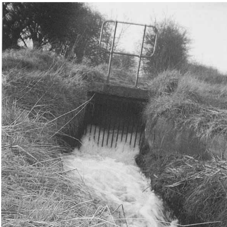
Fig. 4. Outfall of Page Bank coalfield dewatering station (No. 8 on Fig. 1) which pumps about 12 Ml/d into River Wear
