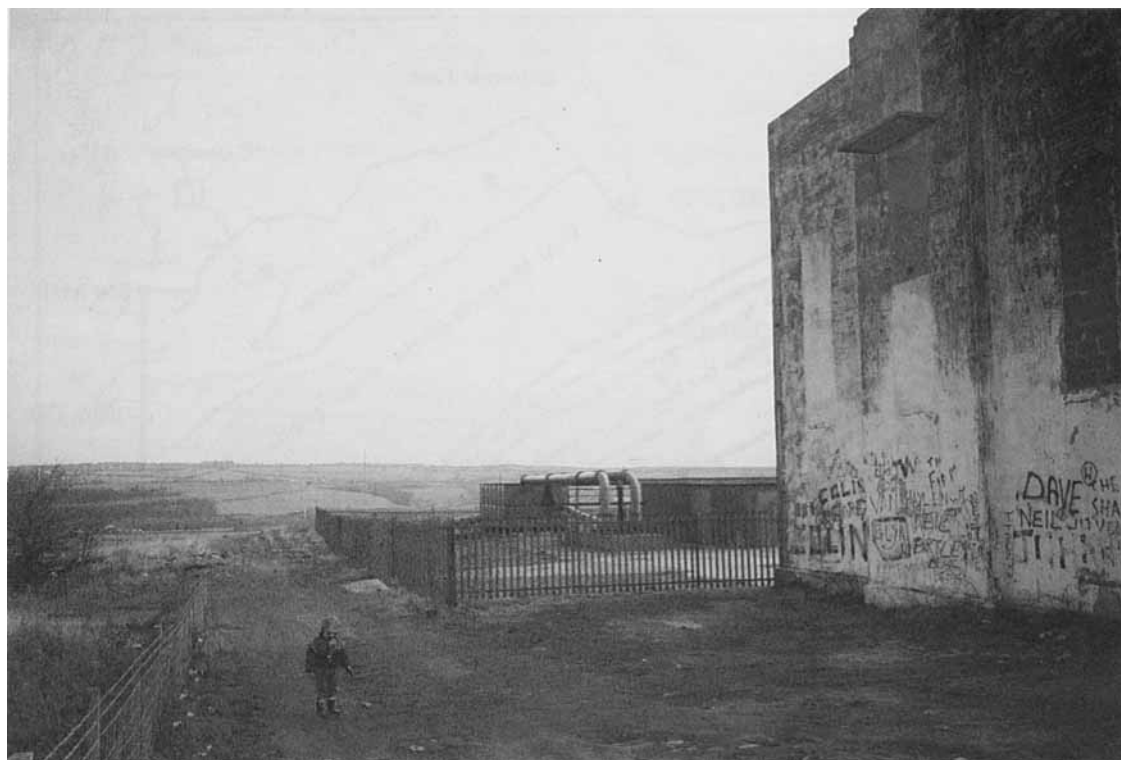
Fig. 3. Kibblesworth Colliery coalfield dewatering station (No. 1 on Fig. 1), Gateshead. Old colliery engine house (to right); twin rising main (pumping 25.7 MI/d) exiting mine shaft and entering header tank (centre of view)
